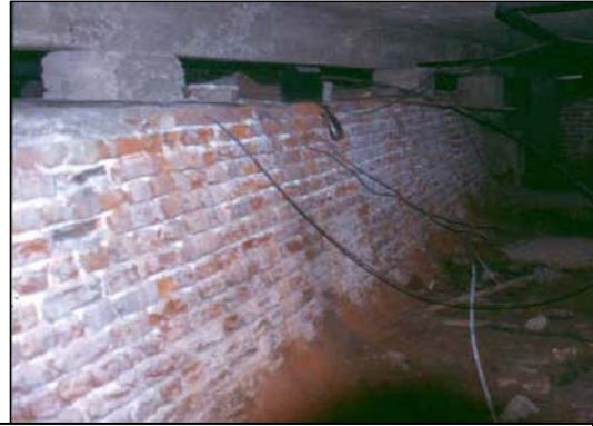
Figure 119: face of Granville Bastion beneath the Missroon House, 40 East Bay Street.
