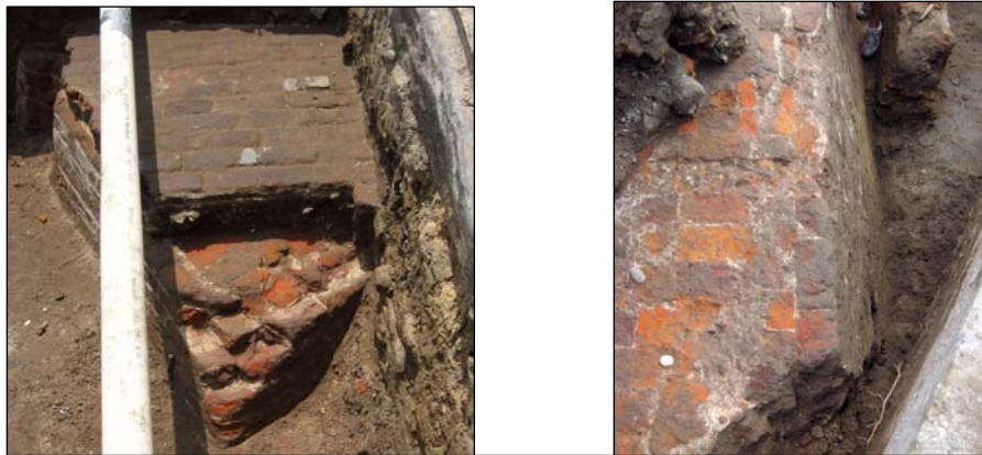
Figure 42: Redan (feature 4) beneath Feature 1; damaged by Feature 9.
