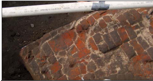
Figure 113: Top of the redan at the point.
