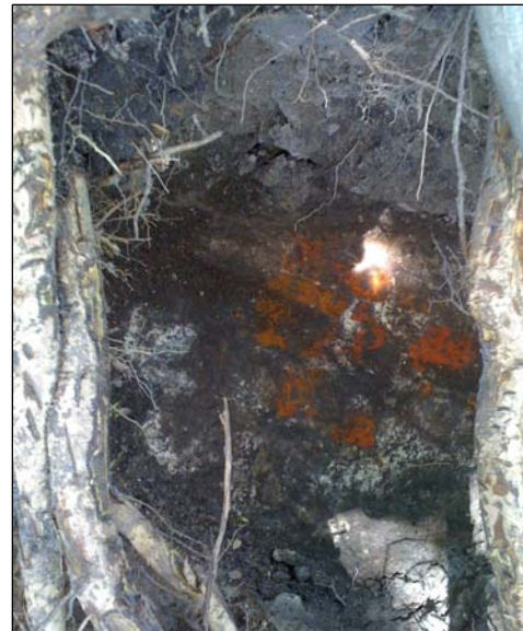
Figure 6: Early brick exposed in construction trench near the kitchen.
