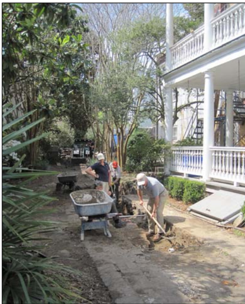
Figure 3: Excavation of area north of wall.
