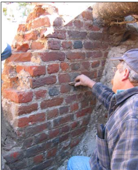
Figure 109: Brickmason Doug Scott.
