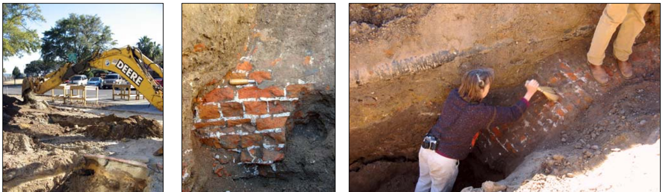
Figure 27: Exposing portion of the redan parapet in Trench 2.
