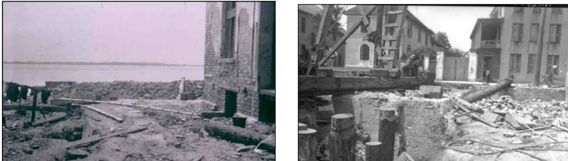
Figure 117: 1920s excavation of Granville Bastion during renovation of Missroom House.
