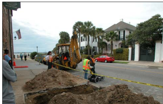
Figure 160: Repairs by Charleston Water Systems guide archaeologists to newly-discovered portions of the wall.
