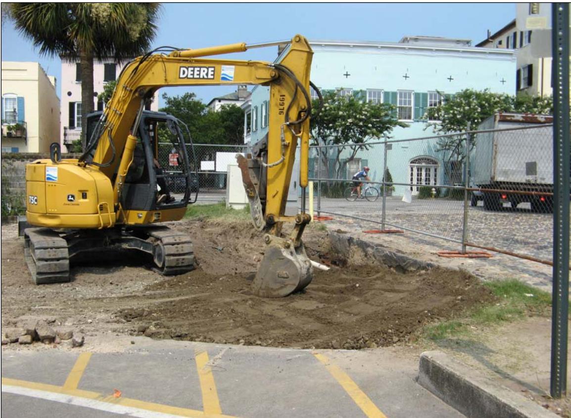
Figure 48: Backfilling of 2009 excavations by Charleston Water Systems.
