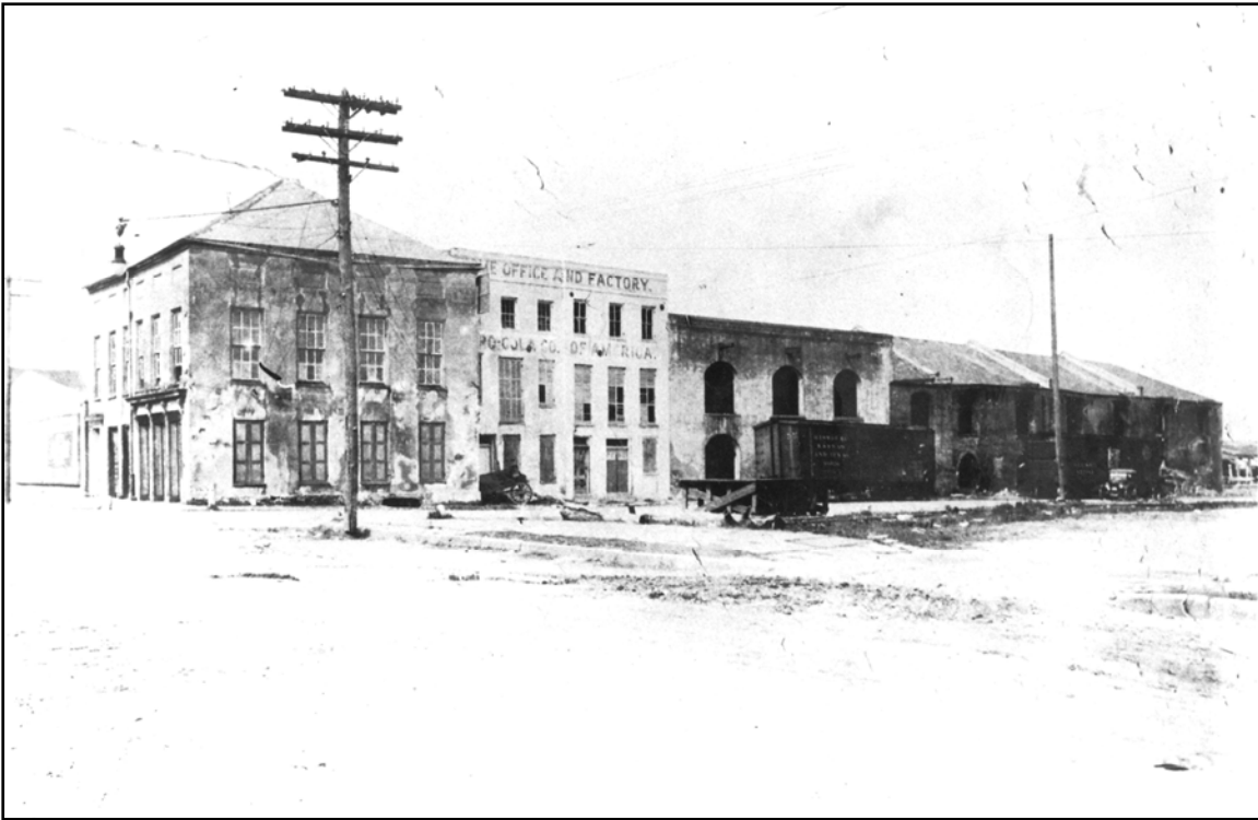
Figure 23: South Adger's Wharf in the early-20 th century. The rail line is visible in front of the range of buildings shown on the 1793 plat, including 90 East Bay Street (courtesy Historic Charleston Foundation).
