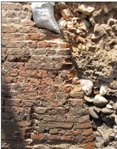
Figure 115: Redan point at base; note the cobble fill.
