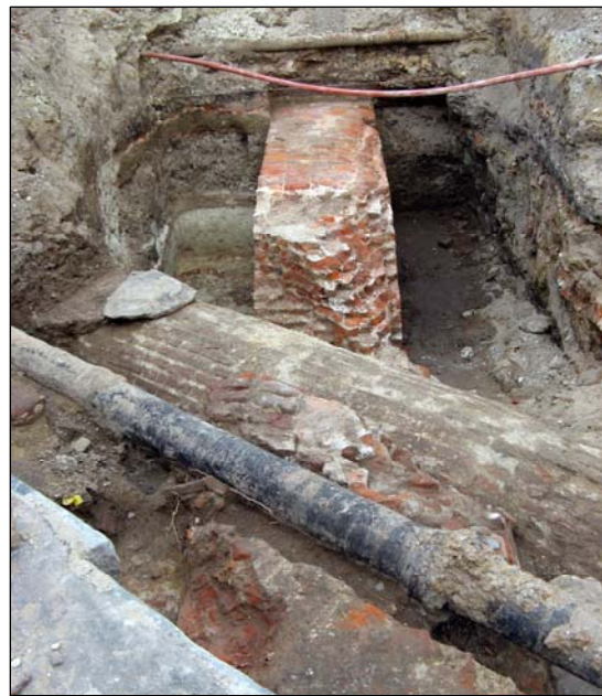
Figure 34: Trench 3, exposing the north face of the redan and Unit 3, exposing the interior, or left, side of the brick.
