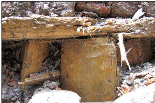
Figure 116: Cypress pile and plank beneath the brick.
